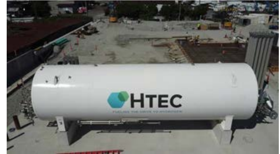
HTEC's liquid hydrogen tank
